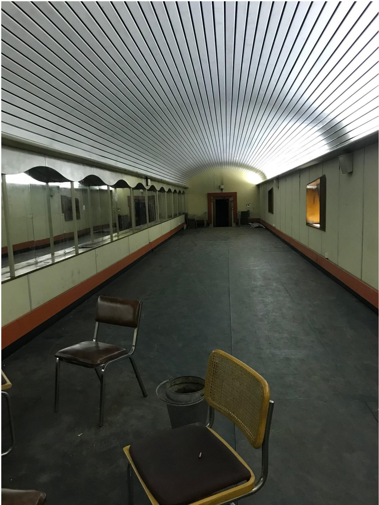
Image 4: Existing canteen with in the Kingsway Tunnels
