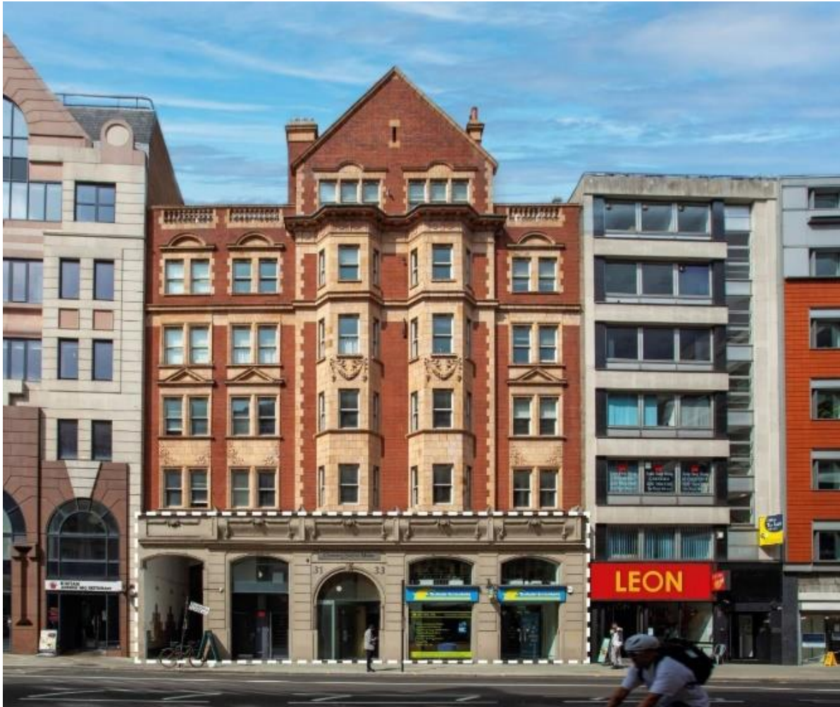
Image 2: View looking north across High Holborn towards 31-33 High Holborn
